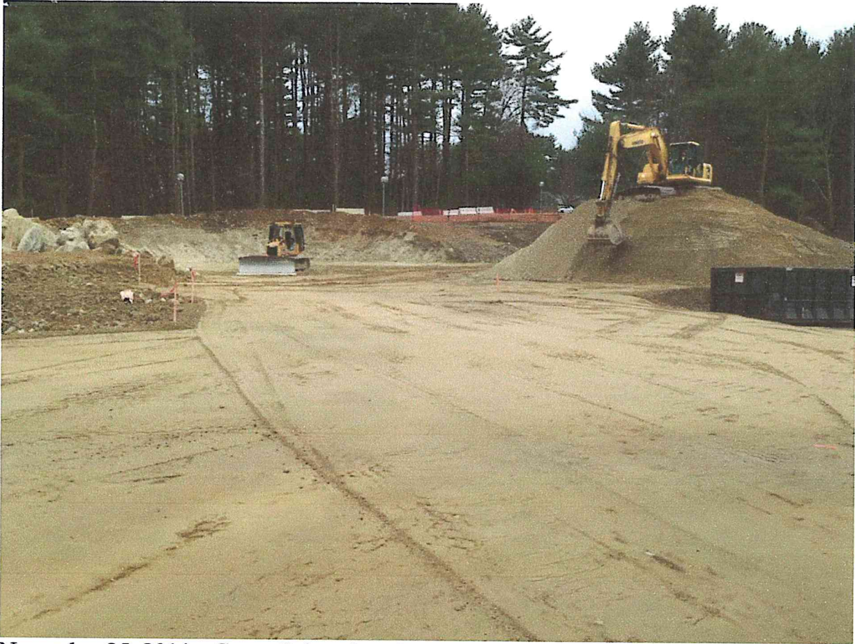
November 25, 2014 – Cut to Subgrade at Rear Parking Area
