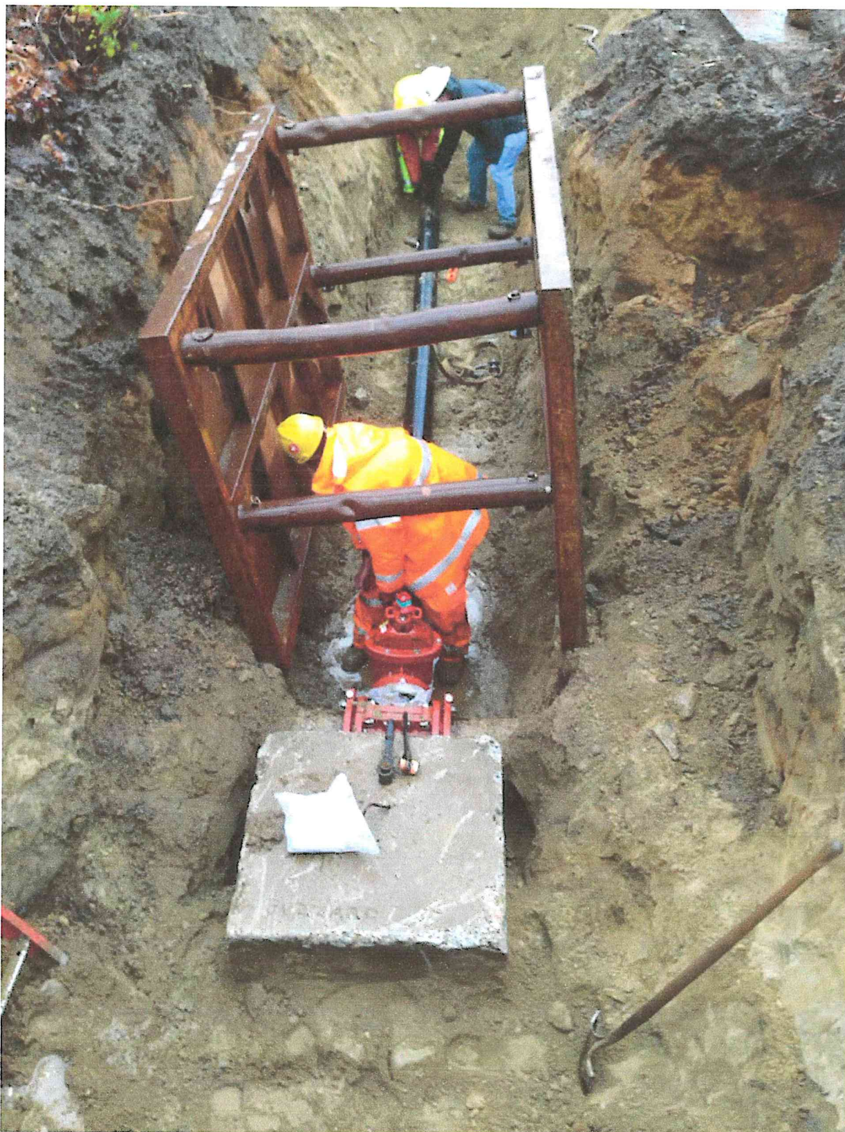
November 17, 2014 – Water Service Connection @ Hudson Road
