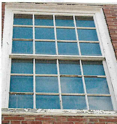
Single pane glass w/o storm windows
